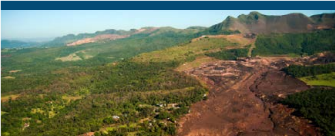
Aftermath of Córrego do Feijão dam collapse | Photo © Ilana Lansky/Shutterstock.com
